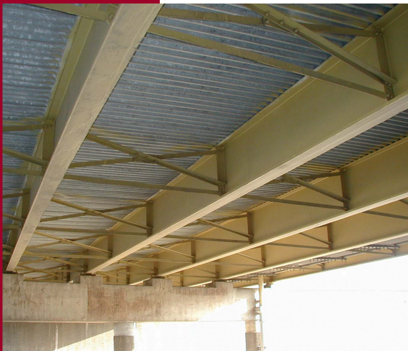
Figure 1 – Typical multi-girder system.
