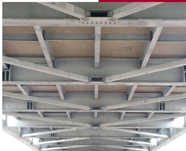
Figure 6 (Above left) – Typical stacked floor system.
