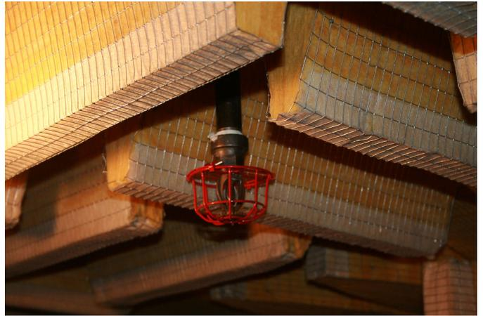
Fig. 9. Anechoic Chamber Fire Suppression
